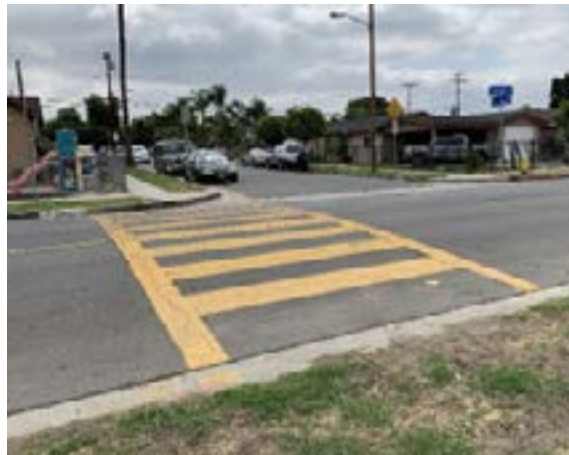
A yellow ladder crosswalk outside of Whaley Middle School on Gibson Avenue
